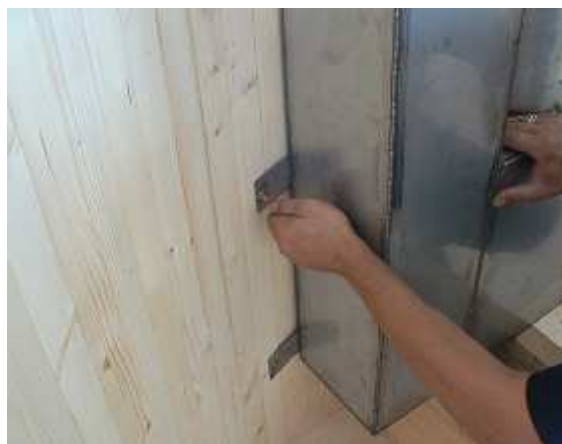
Foto 12. Mark the center of hole
