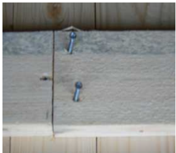
Photo 2. Screwing screws into the bottom boards
