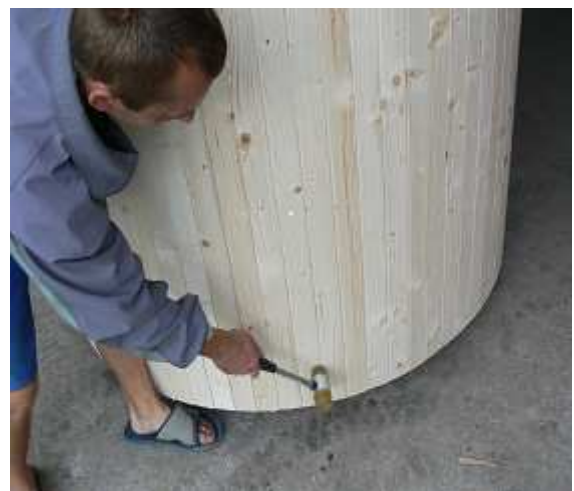
Photo 6. Tap the slats over once more when finished
