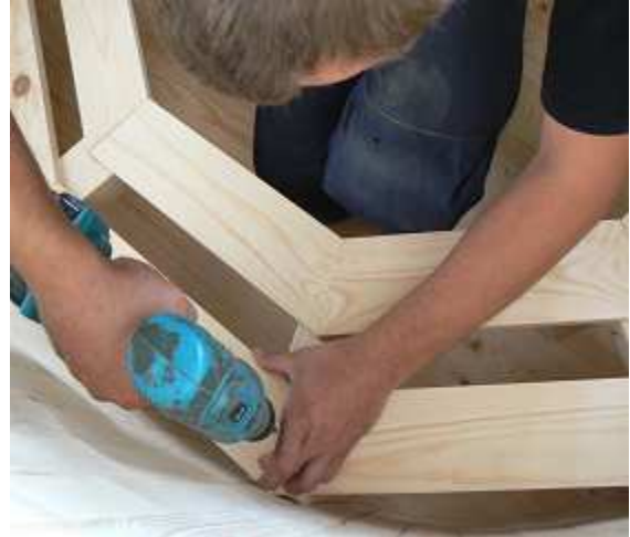
Photo 16. Fastening of the sitting boards
