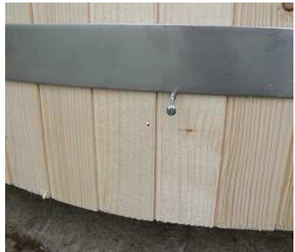
Photo 8. Hoop resting on the screws
