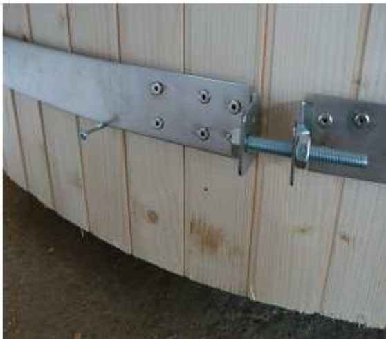
Photo 9. Fastening of the tightening bolt
