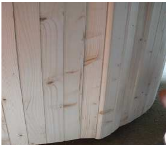
Photo 5. Positioning the last slat
