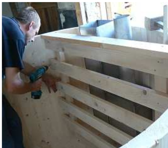
Photo 14. Positioning of the grate
